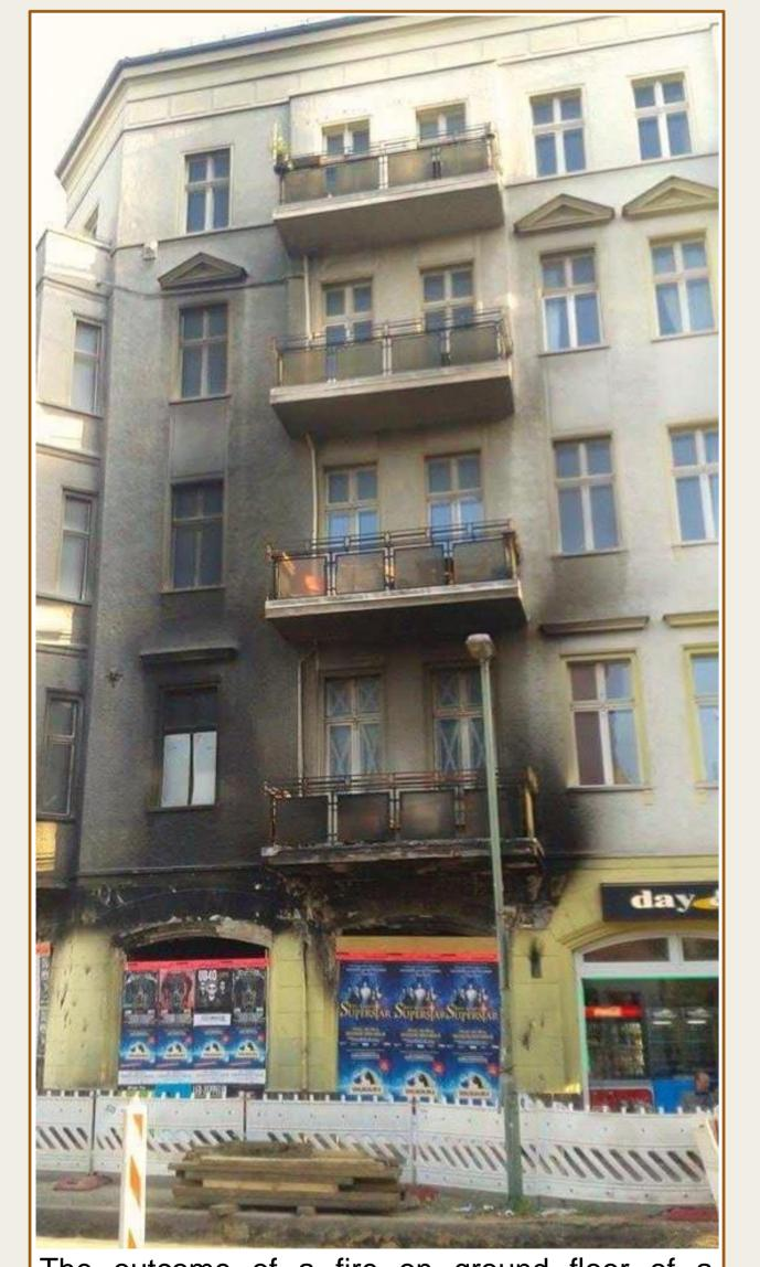
The outcome of a fire on ground floor of a residential building in Berlin. In this case the use of horizontal projections (right) resulted in less consequences on the facade compared to a vertical safety distance (left), as seen on the smoke damage and broken windows.
