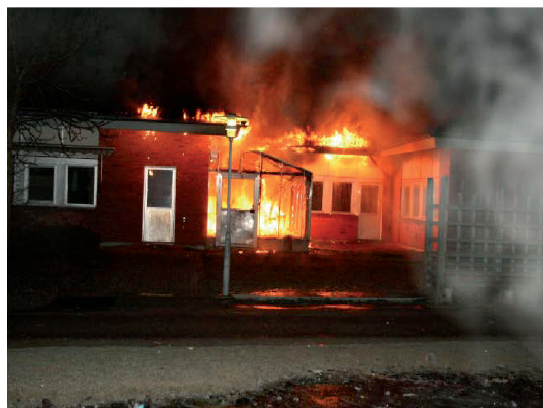
A typical fire scenario that causes great monetary loss. A fire is deliberately lit outside the school building and has spread to the roof and attic of the school. The fire was devastating and 2/3 of the school was destroyed in the fire.
