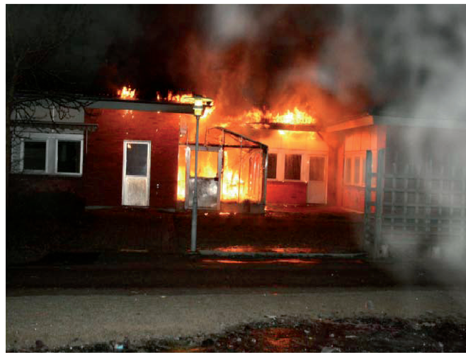
Figure 2: A typical fire scenario that causes great monetary loss. A fire is deliberately lit outside the school building and has spread to the roof and attic of the school. The fire was devastating and 2/3 of the school was destroyed in the fire.
